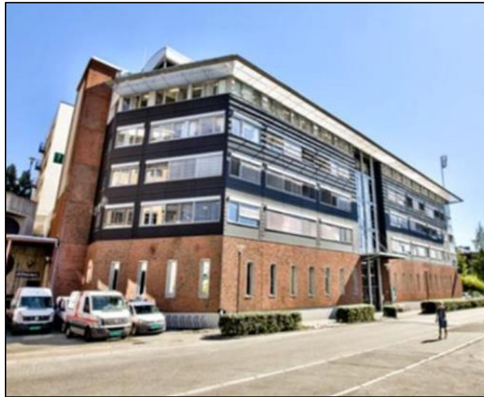
Oncoinvent has in-house GMP production capability
